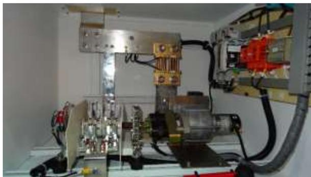
**Older 8800261 Contactor Panels had external Bonding Devices 858961 & 863118**
