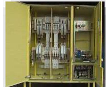
4.29 MLU CWRS – 2 Pole Remote Controlled Wash Road Contactor - 3200A 630V DC -
