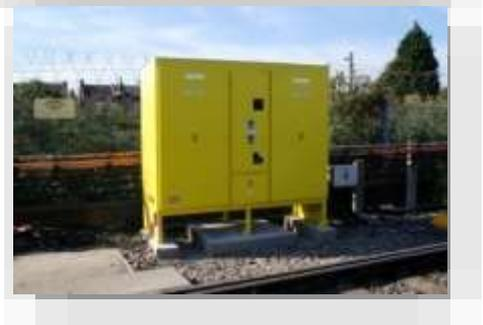
**4.27 MLU MCOID - 2 Pole Manual Changeover Off load Disconnecter 4000A 630V DC -**
