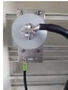
The Gosforth Depot Protection Isolator consists of a 2.0kA 1.5kV Disconnecter in a bespoke enclosure.
