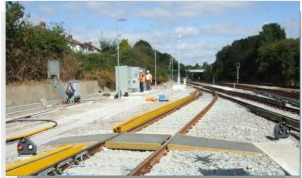
A monitoring system for Insulated Block Joint Failure is incorporated in the Mechanically Operated Buffer Zone Panel to ensure that the insulation between Traction Negative and Depot Earth is maintained.
