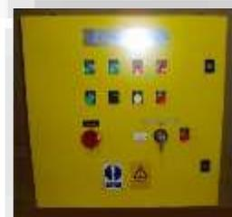
**6.17 MLU RCTIS Remote Controlled Track Isolating Disconnecter Switch (Tunnel) 4kA 2 P Slimline 8800411**
