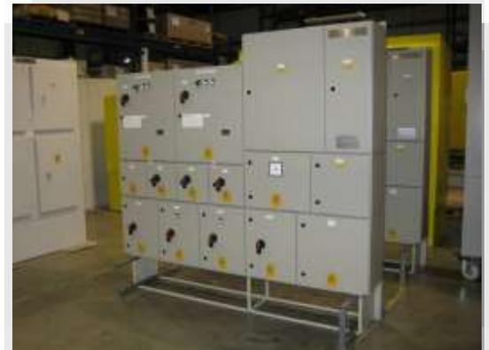
**15.6 LVAC 3 Panel Switchboard – 100A 400/440V AC 3ph 4 Wire - Network Rail No PA05/02022 - 8800382**
