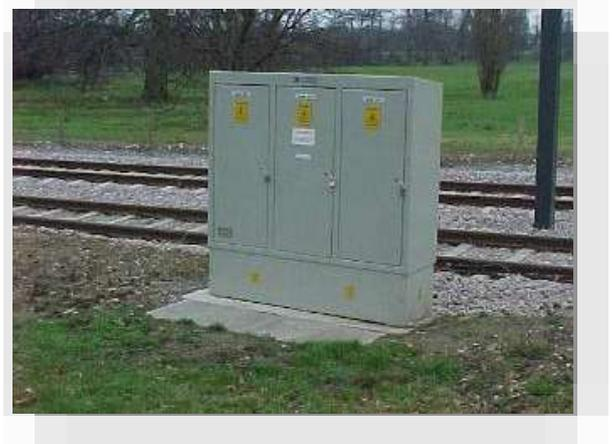
**2.8 TL RCTIS– 2 Pole Remote Controlled Track Isolating Switch – 2000A 750V DC - 8800387**
