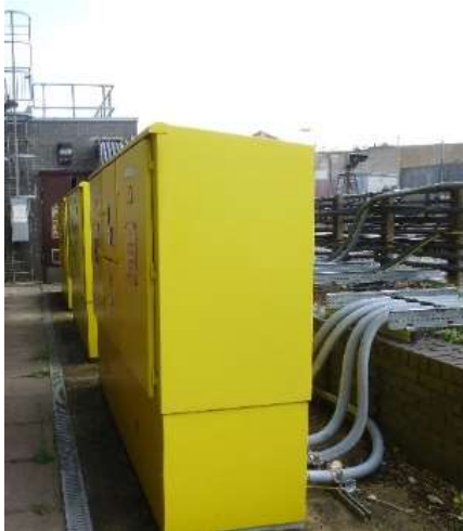
2 pole Track Disconnectors on London Underground
