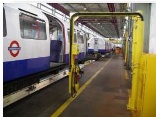
Overhead Boom in use
